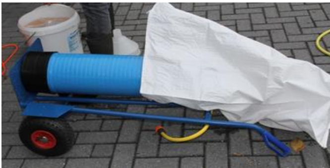
3. lay the trolley flat, allowing the resin from the bottle (including water) to drain into the bag
